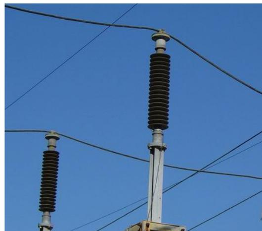
Figure 1 The SIR insulators under study
