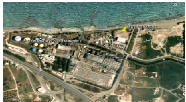
Fig. 4. A view of the Linoperamata Substation
