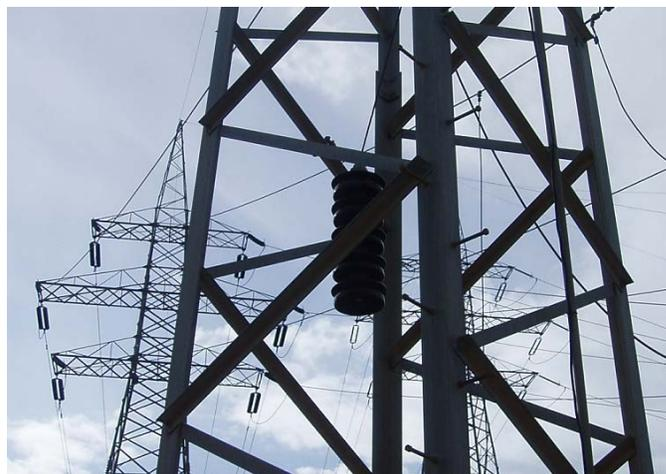
Fig. 6 Offline installation of an insulator string for ESDD measurements
