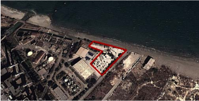
Fig. 6. The location of TALOS High Voltage Test Station
