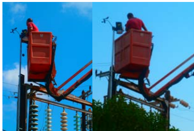
Figure 7. Installation of the weather station in top of the ESDD arch
