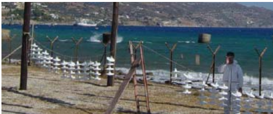
Figure 3. HEDNO personnel coating suspension insulators with RTV SIR
