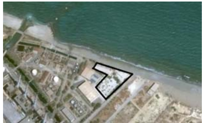
Fig. 9. The location of TALOS High Voltage Test Station
